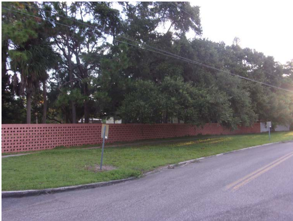
VIEW OF SUBJECT PROPERTY FACING NORTHEAST FROM 22 ND AVENUE
