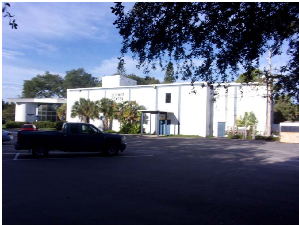
EASTERN ELEVATION FACING SOUTHWEST
