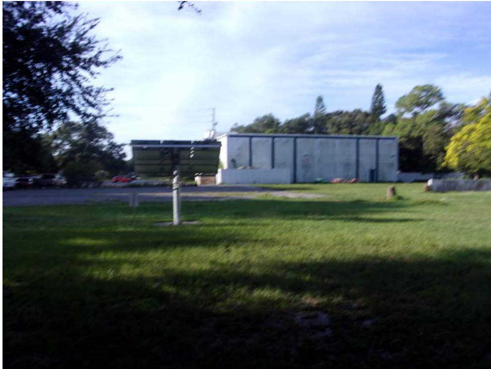
REAR OF STRUCTURE FACING SOUTH
