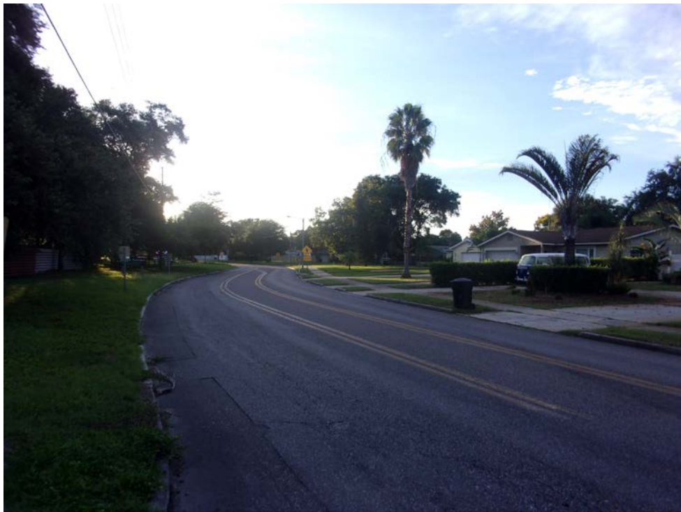
22 ND AVENUE FACING EAST SUBJECT LOCATED ON LEFT SIDE OF PHOTOGRAPH
